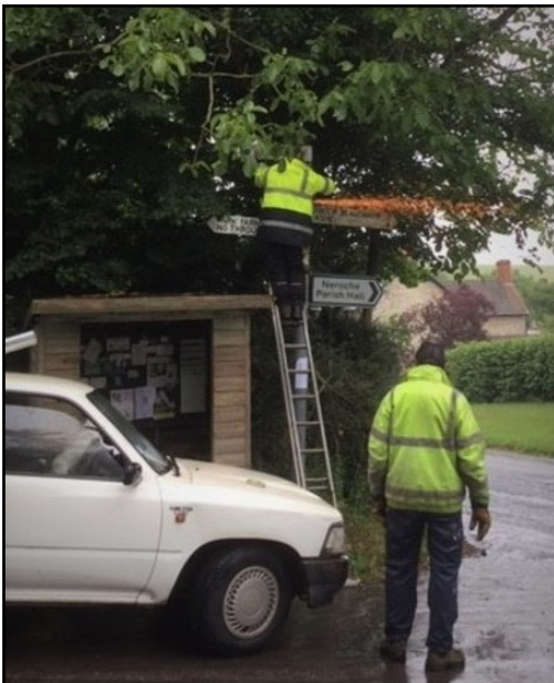
Somerset Forge dismantling the post
