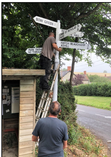
Somerset Forge reassembling Staple Fitzpaine Fingerpost
