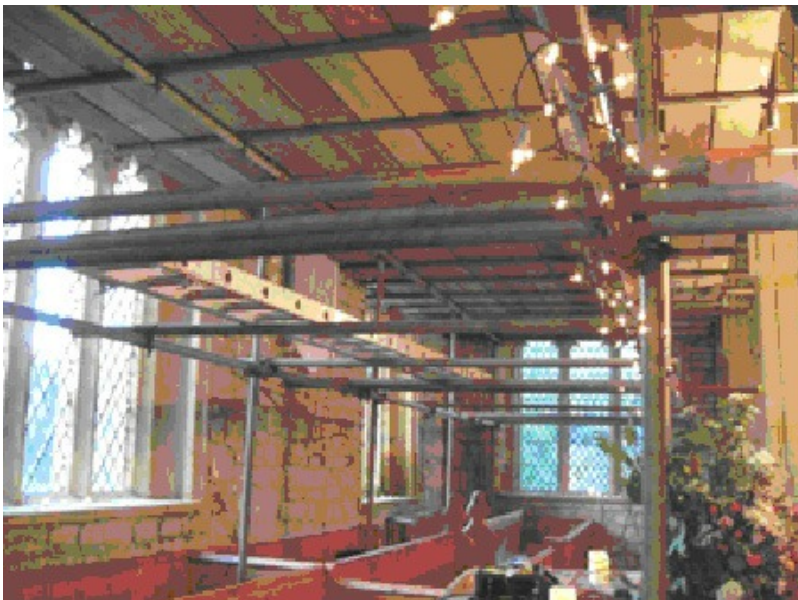
St Peter's roof under repair
